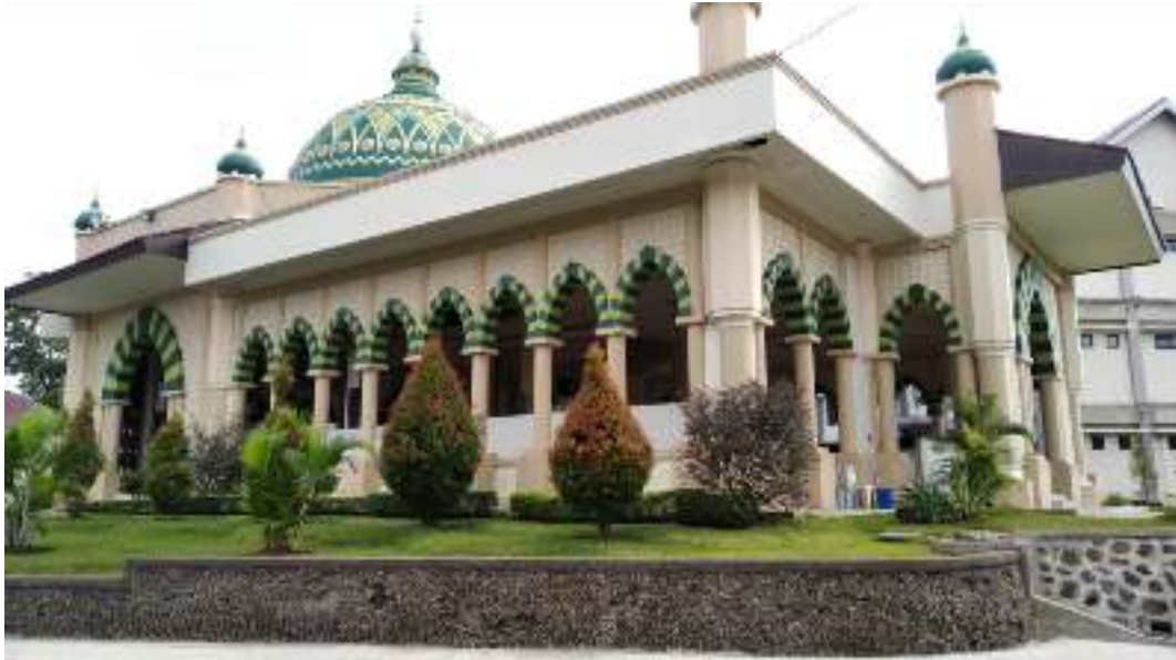
MASJID SUCHARY DI KAMPUS ISTIQOMAH SAMBAS BOARDING SCHOOL PUTRA PURBALINGGA TAMPAK LUAR
