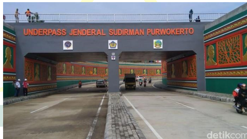
Gambar 3. Underpass Jenderal Sudirman
